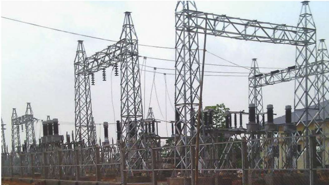
66/33kV, 10MVA Substation(Under Construction) 65(T)/ESE/2014-2015
