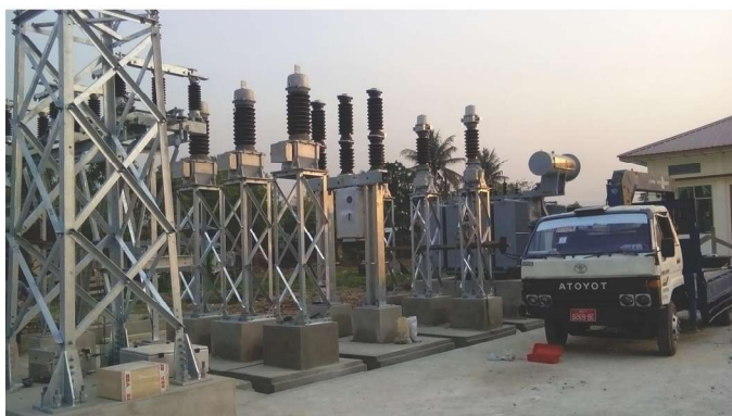
33/11kV, 5MVA Substation(Under Construction) 111(T)/ESE/2014-2015
