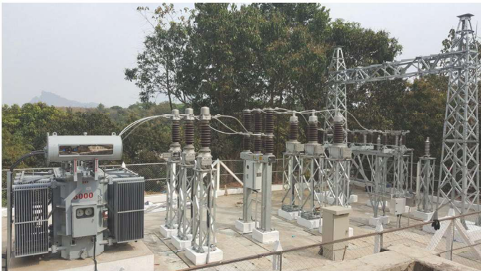
33/11kV, 5MVA Substation(Under Construction) 65(T)/ESE/2014-2015
