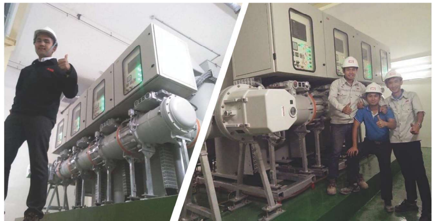
Junction City from Shwe Taung Development Co., Ltd. 66 kV & 11 kV GIS Substation
