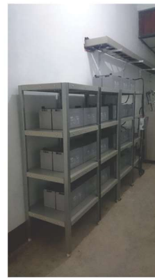
UPS Power Wave 33, 12 SP 120 FR, 1x42x120AH, 42 no.
