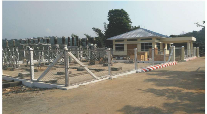
33/11kV, 5MVA Substation(Under Construction) 65(T)/ESE/2015-2016
