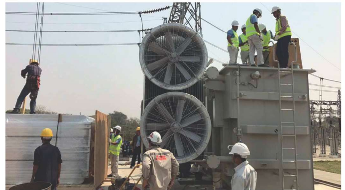
230/33/11 kV, 100MVA, Three Phase Transformer Installation in 2017
