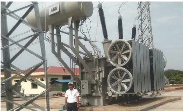
230/33/11 kV, 100MVA, Three Phase Transformer Installation in 2017
