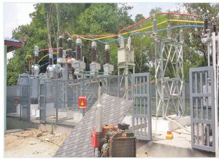
33/11KV Substation Aggregate Mining Plant @ Mon State
