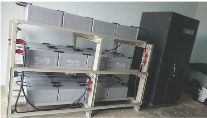
UPS Power Wave 33, 12 SP 120 FR, 1x48x120AH, 48 no.
