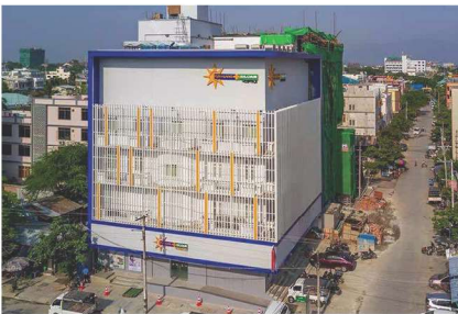
230/400V Low Voltage Distribution Panels From PUNHLAING SILOAM Project
