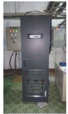
UPS Power Wave 33, 12 SP 120 FR, 1x42x120AH, 42 no.
