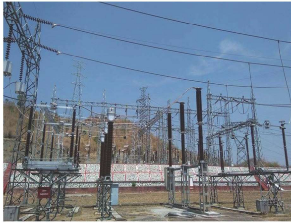
245kV, Gas Circuit Breaker @ Shwe Taung Substation
