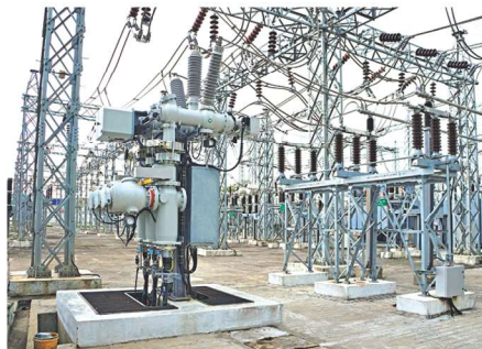
72.5 kV HGIS for Ahlone International Port Terminal @ 230 kV Ahlone Substation
