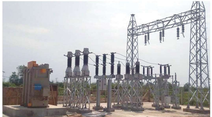
66/11kV, 5MVA Substation(Under Construction) 9(T)/ESE/2015-2016
