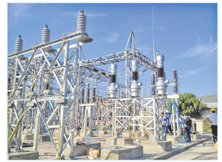
36 kV Switchbay extension @ 230 kV HlaingTharyar Substation
